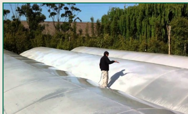
FIGURE 3: Manual whitewash application
