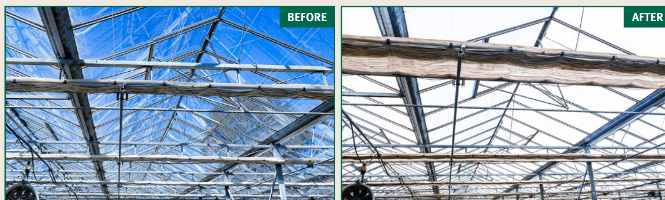
FIGURE 8. Before / After Results of Whitewashing with Drone
